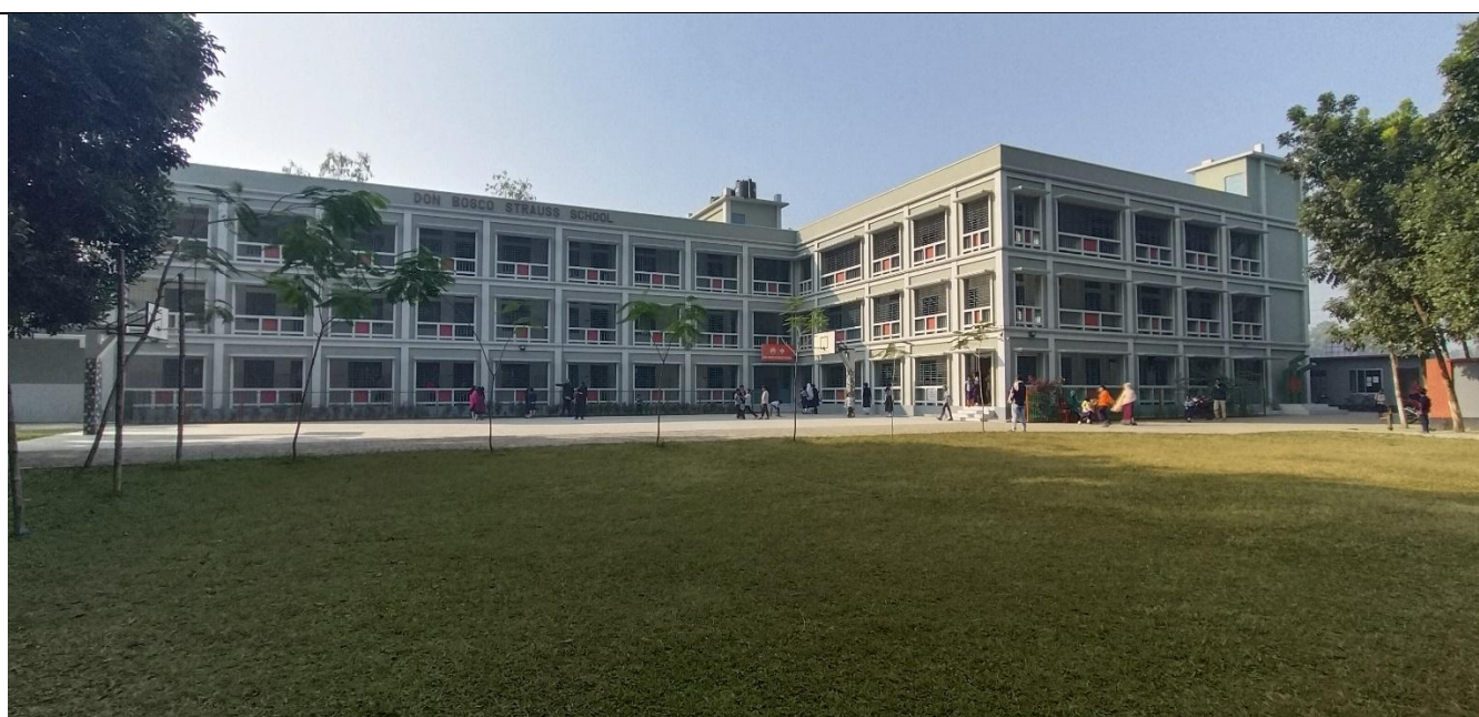
Don Bosco Strauss School Building, Khanjonpur, Joypurhat, Rajshahi.
